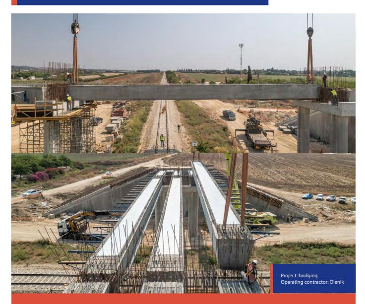
Prestressed beams use allow to reduce the cross-sections of members and the weight applied to the building (vs. conventional beams).
