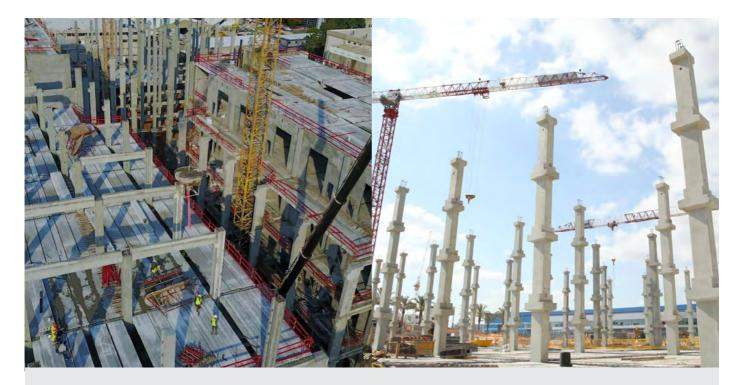
Ramet Tron specializes in the design and manufacture of tall precast concrete columns of up to 20-m and more, of variable cross-sections. The columns are manufactured in accordance with the customer's instructions, according to their needs and the building's purpose: swimming pools, stadiums, logistic and public centers, offices, water desalination plants and many other applications.
