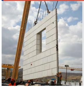
The manufacture of precast elements by dedicated plants offers numerous advantages to the operating contractor and/or entrepreneur (the customer). Firstly, the manufacturing process is conducted using customized precision steel forms, allowing to manufacture a high volume of elements of various types (according to the project's requirements).
