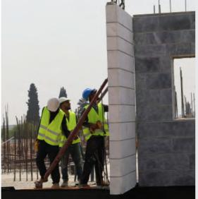
Precast construction allows to maintain a well-planned, neat and orderly construction site. Therefore, the time required to complete frameworks can be significantly reduced, as the assembly of precast elements and members is conducted in advance.
