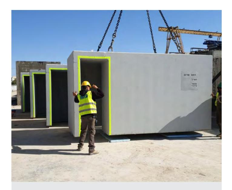
Transportable Moovable Room shelters approved by the Home Front Command provide a protection solution equivalent to that manufactured on site, therefore they offer a valid alternative, when a protection solution is required.
